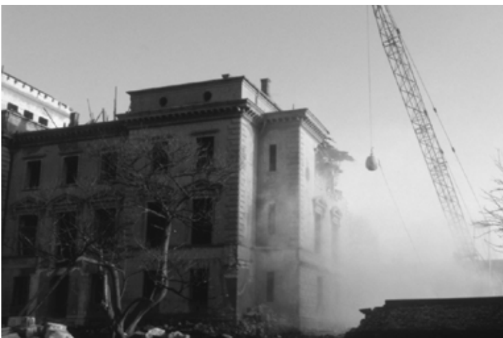
The demolition of the castle
